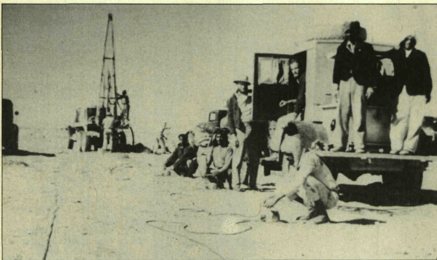
An early seismic crew works near Abu Hadriya, circa 1939. The man in the foreground is planting an S-10 seismometer weighing 10 pounds. "That was considered quite an improvement over the way we started in 1930, with S-2 seismometers weighing 30 pounds each," said Green. Today's seismometers weigh "about a fraction of an ounce." (Courtesy, C. Green)
